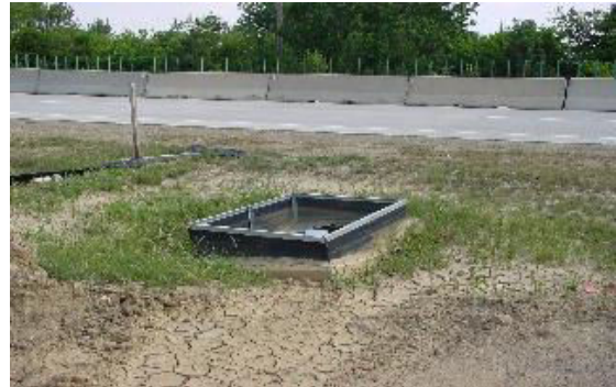
ODOT # 4 Multi-Angle Bar Grate VERTIPRO® INTERSTATE 270 RECONSTRUCTION, GROVE CITY, OHIO
