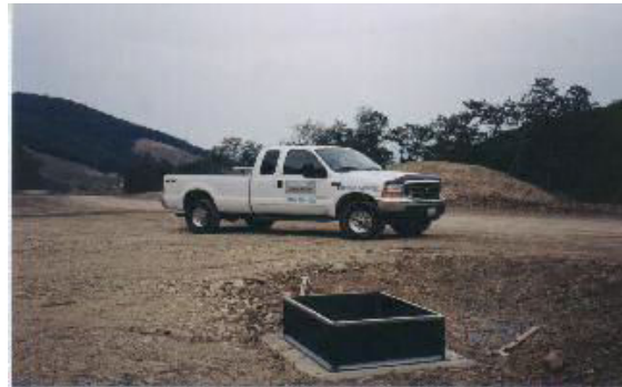
WVDOT # 750 VERTIPRO® Corridor H - Baker, WV
