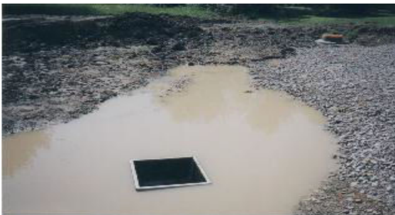
Virginia #3030 - 30" x 30" x 16" h VERTIPRO® Immediately following a rain storm
