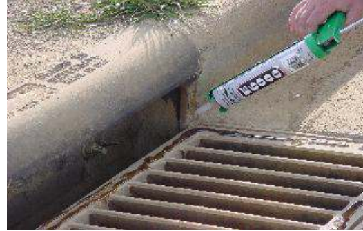
#2. APPLY BEAD OF E-6000 ADHESIVE TO GRATE
