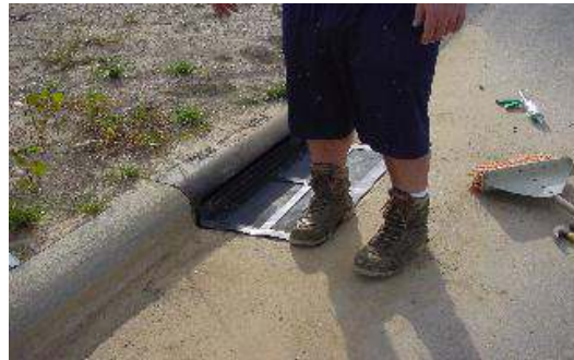
#4. STEP ON SLAMMER® TO EVEN OUT ADHESIVE. THAT'S ALL THERE IS TO IT!
