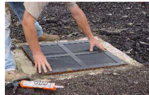
#4. PRESS GrateFX® INTO PLACE TO EVEN OUT ADHESIVE. THAT'S ALL THERE IS TO IT!
