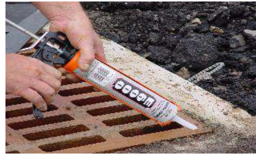
#1. APPLY BEAD OF E-6000 ADHESIVE TO GRATE
